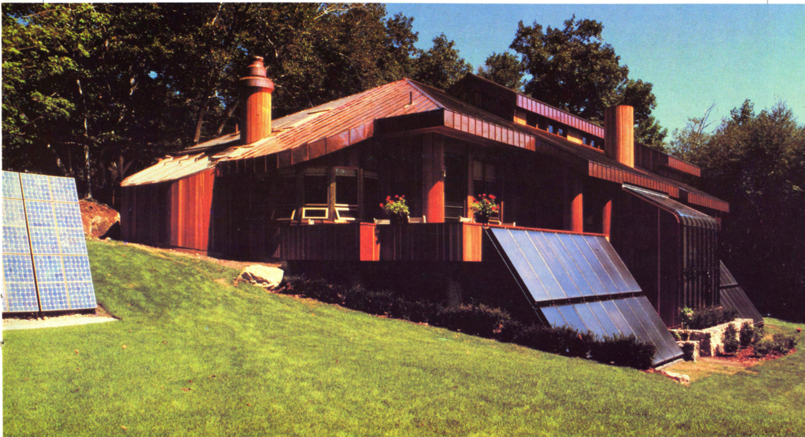
This view of the south, energy-producing side of the Sun/Tronic House shows part of the 150-square-foot photovoltaic array, which provides part of the electrical needs for the home.
