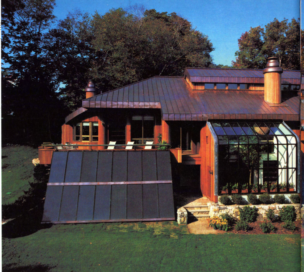
The home's rear view is dominated by the huge solar waterwalls and greenhouse/solarium.
